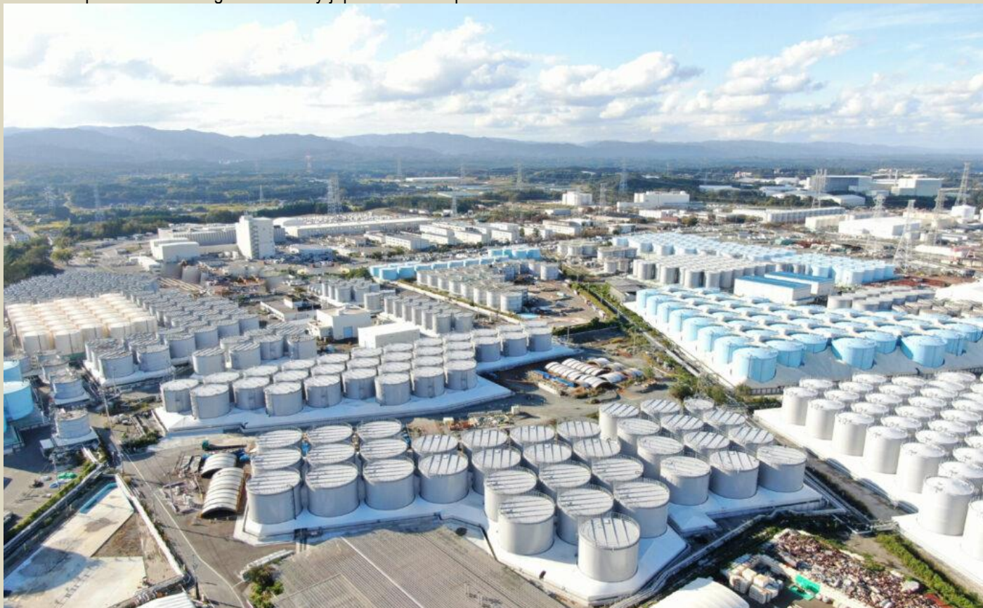
Water tanks holding contaminated water at Fukushima Daiichi nuclear power plant in Japan. (Credit: IAEA)
