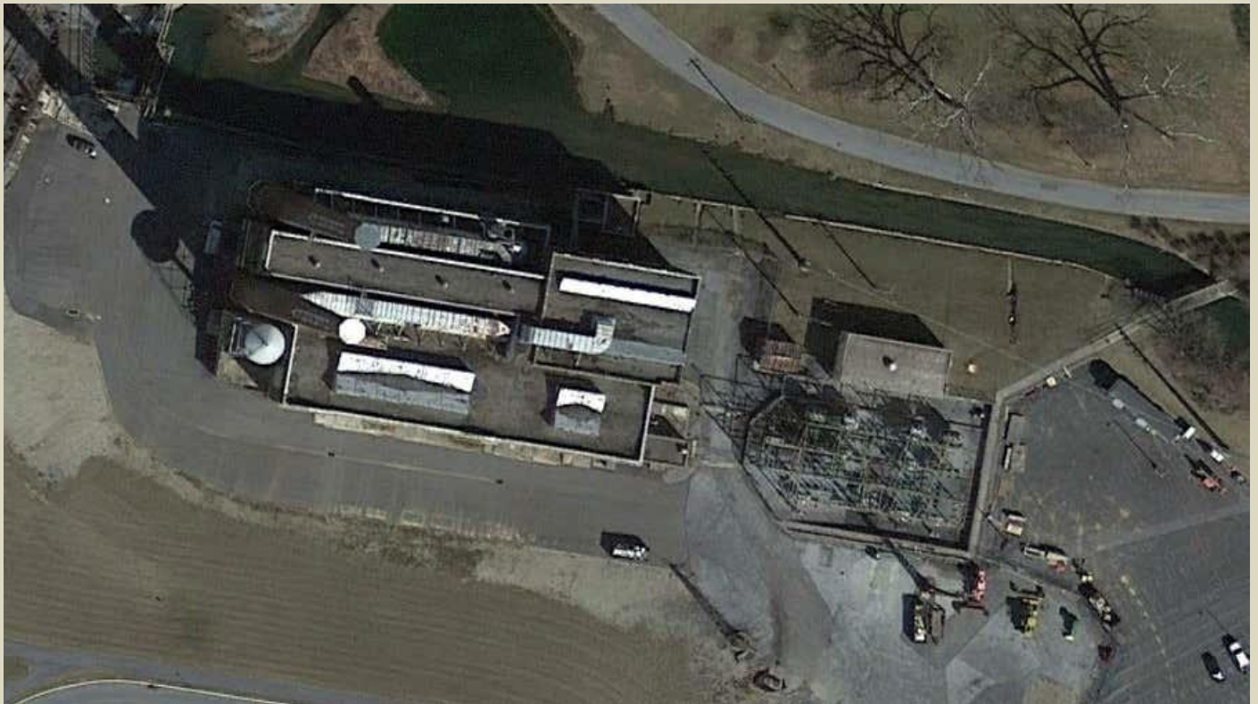
A closer view of the substation and adjacent building where the drone was recovered last year.
