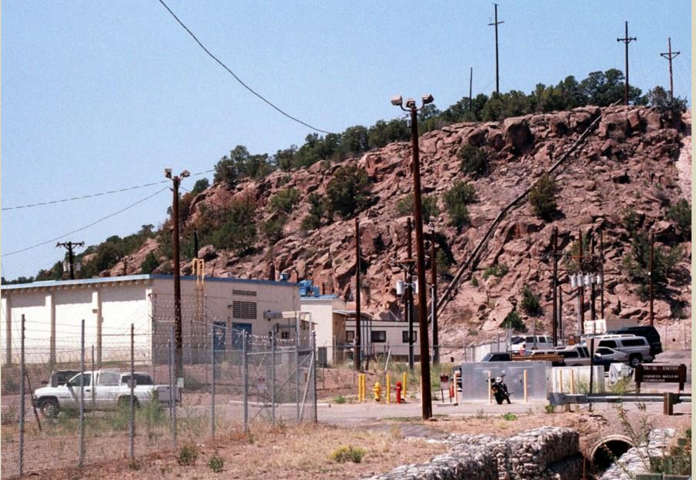
Technical Area 18 of the Los Alamos National Laboratory, which houses several tons of highly enriched uranium and plutonium, and is located at the bottom of a canyon, is shown August 12, 2002, in Los Alamos, N.M. The topography has led critics to say the site is indefensible. (Photo by Neil Jacobs/Getty Images)
