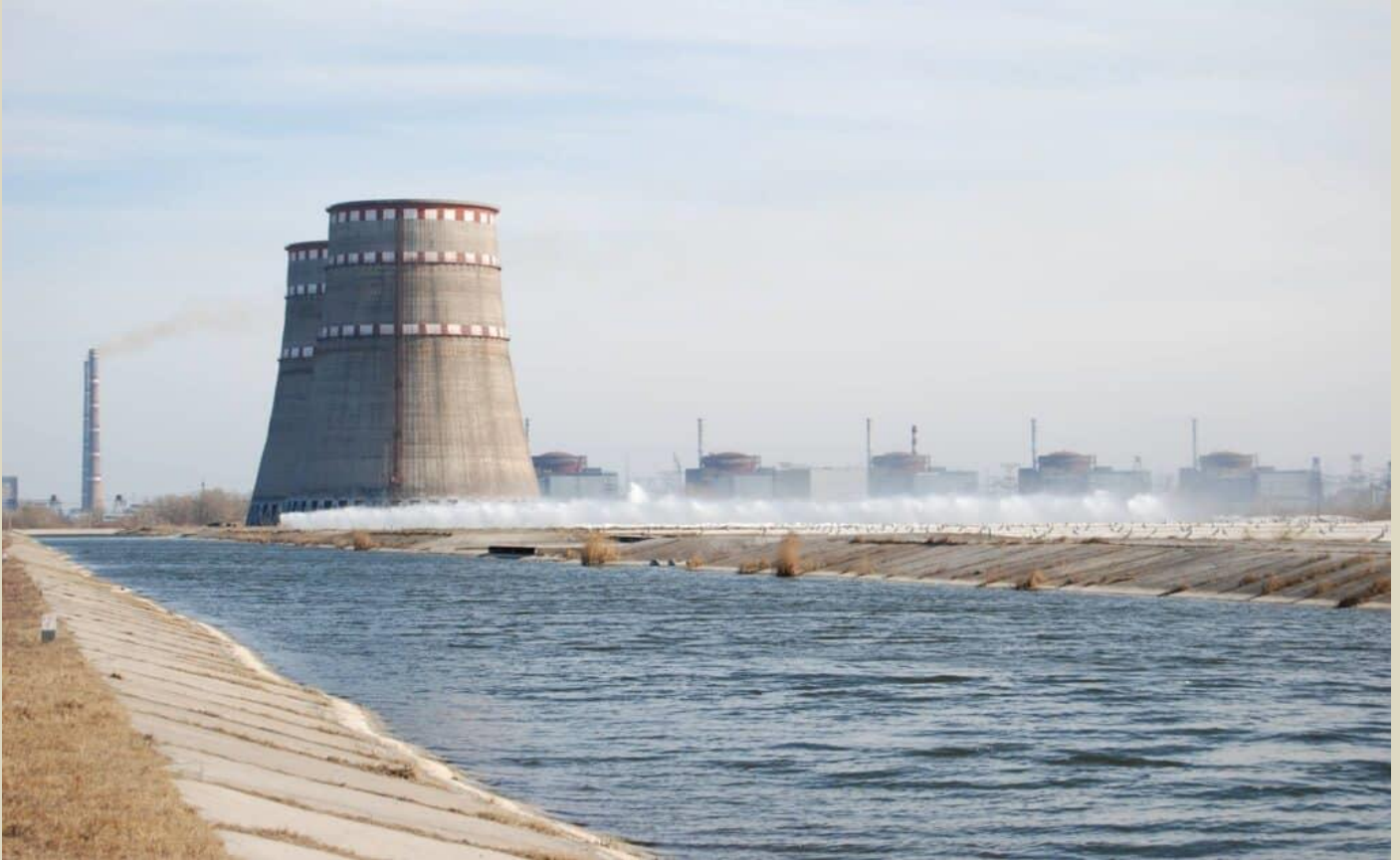
Cooling spray ponds, cooling towers, and reactor buildings at the Zaporizhzhia nuclear power plant. (Photo: Energoatom)
