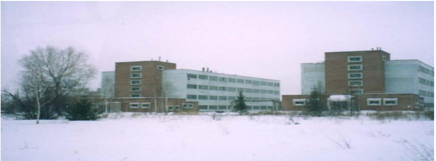
Smallpox Repository (building on right) at the Vector Research Institute, Koltsovo, Russia. (GAO)
