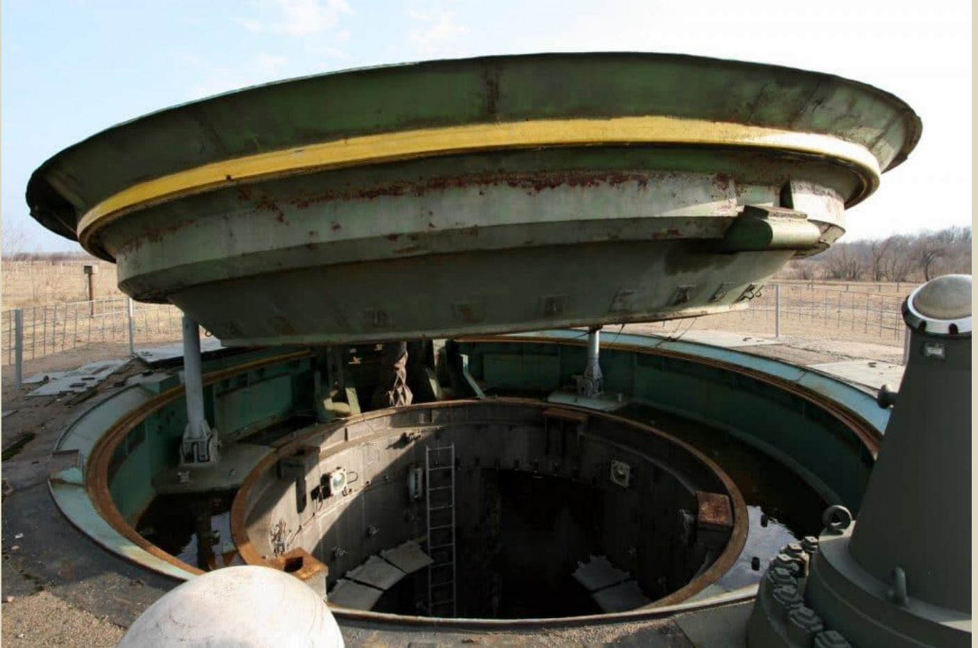
(Rusted) Missile silo of a SS-24 missile, Strategic Missile Forces Museum in Ukraine. Credit: Michael. CC BY 3.0. Accessed via Wikipedia.
