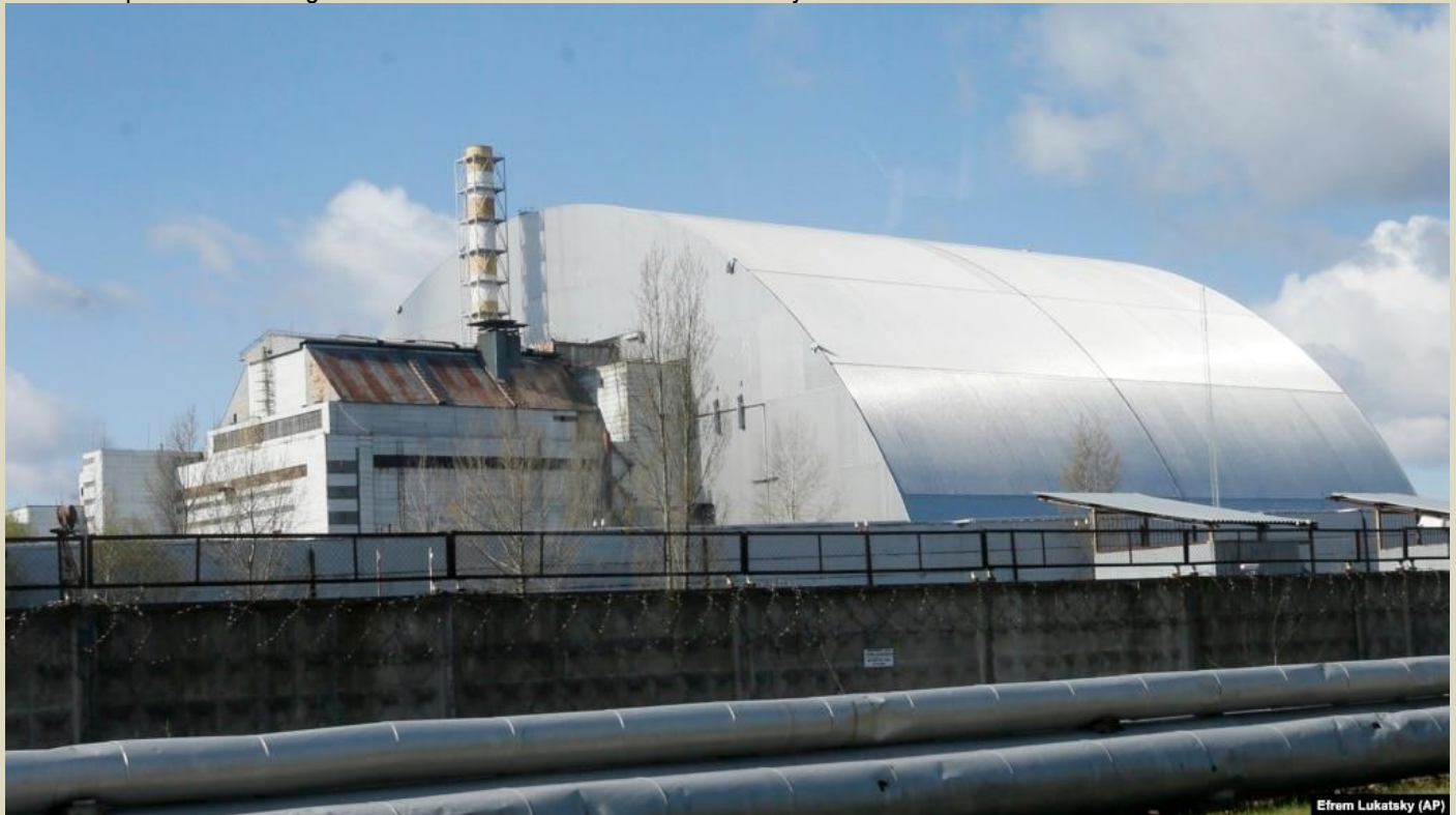
A shelter construction covers the exploded reactor at the Chernobyl nuclear plant, in Chernobyl, April 27, 2021
