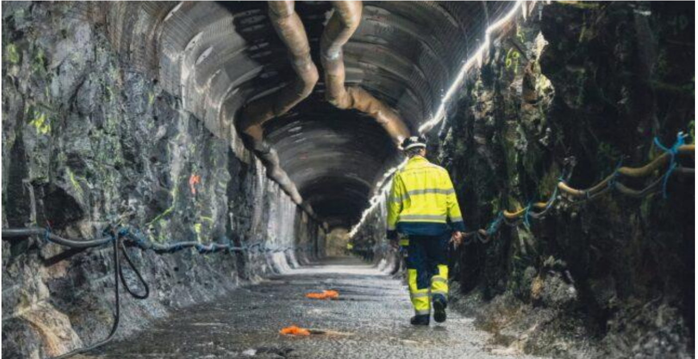
An underground tunnel leading to Finland's Onkalo nuclear repository. (Alessandro Rampazzo/AFP)
