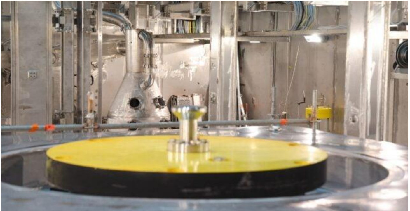
The 'hot cell' fuel handling chamber at the encapsulation plant of nuclear waste management company Posiva. (Alessandro Rampazzo/AFP)
