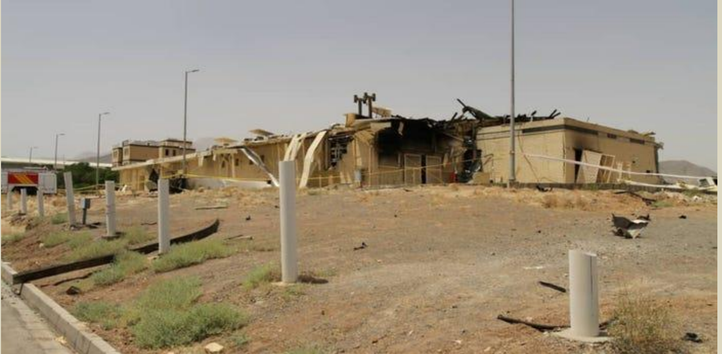
A damaged building after a fire broke out at Iran's Natanz nuclear facility, in Isfahan, July 2, 2020. Reuters
