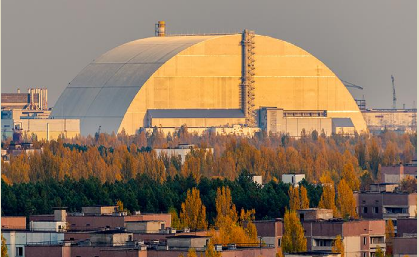
A 'sarcophagus' over the top of the remains of Chernobyl block 4. (Robert Ruidl/Getty Images)
